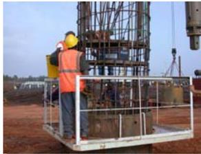
Installation of O-cell arrangement and cage within the pile
