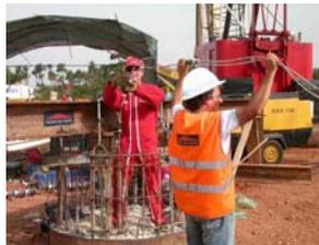
Installation of one of the removable extensometers
